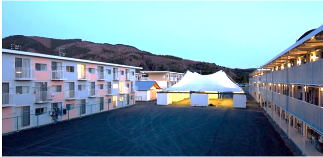
Figure 6. Container Temporary Housing, Onagawa, Miyagi Prefecture
