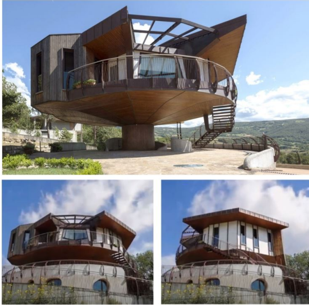
Figure 5. 360 degree rotating house, Roberto Rossi's residential project in Italy (URL-3)
